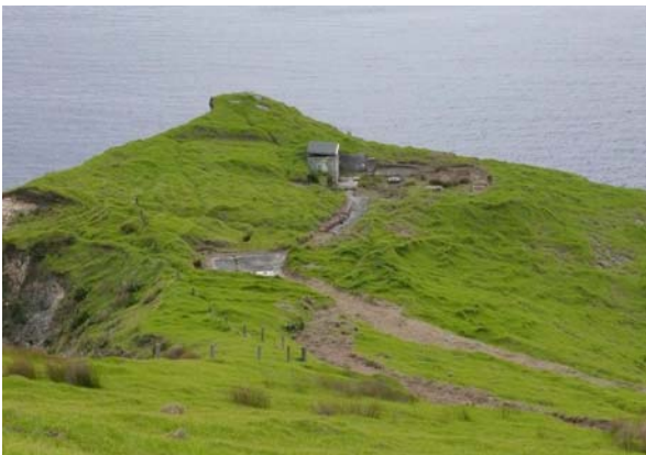
The cleared area around the first house and power house.
